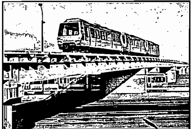
Automated Guideway Transit (AGT) circulating within Chicago's O'Hare Airport terminals and parking.
